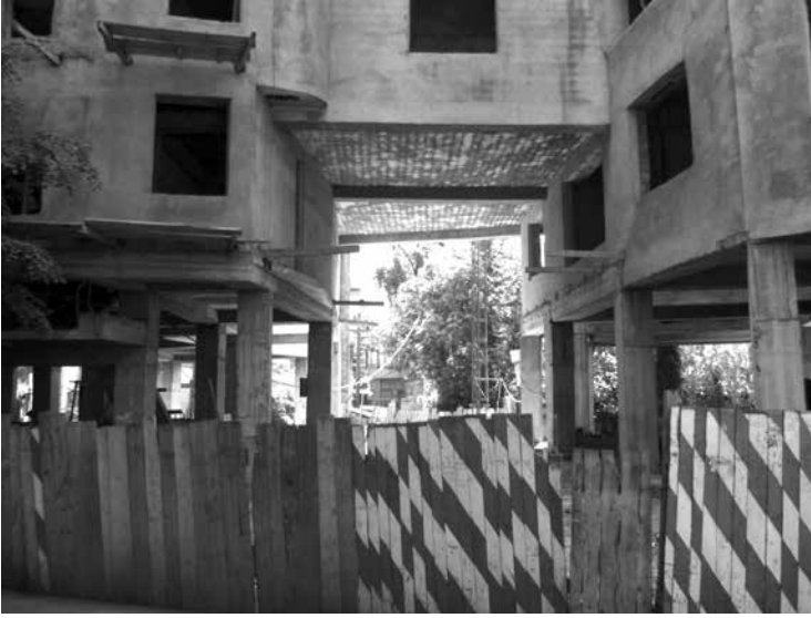
PICTURE 5 Rodin Street closed by construction and arch passage
