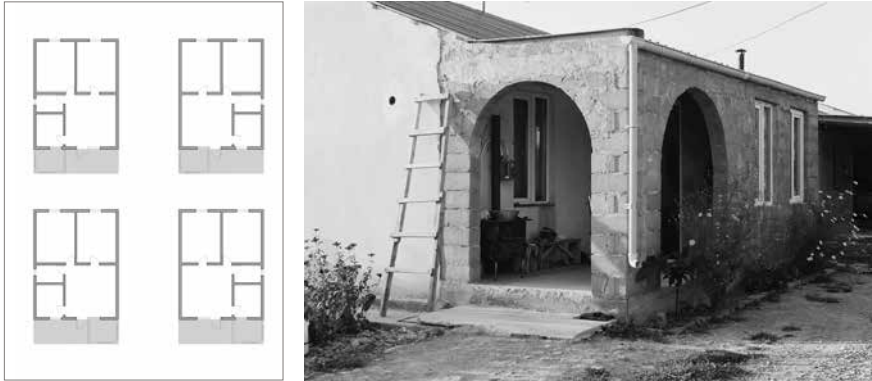
PICTURE 5 Alterations of front façades - Combination of open porch and closed space
