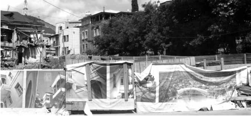
PICTURE 1: Images around the demolished site.
